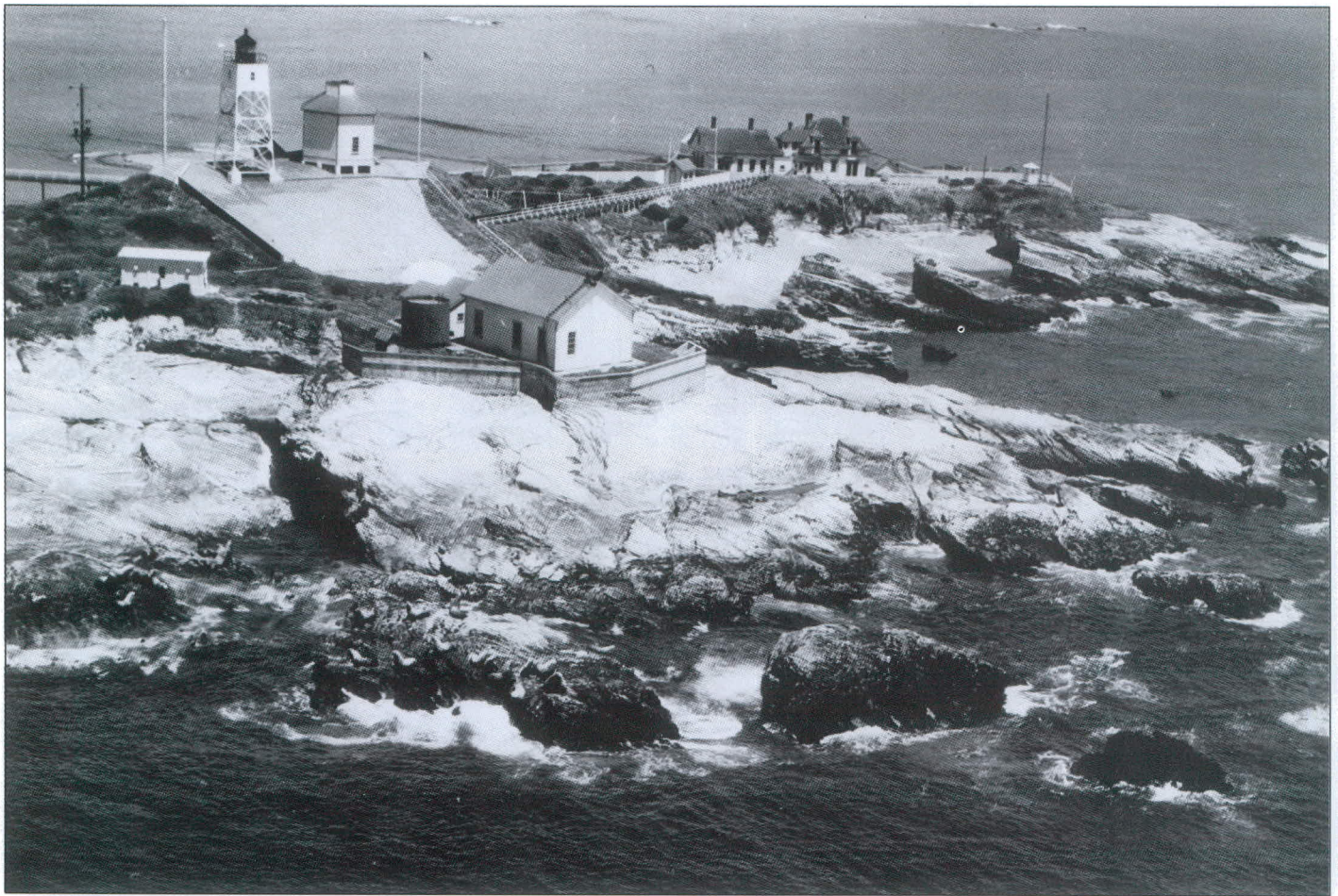
Above— The Año Nuevo Island station began as a fog signal station, a light wasn't installed until 1900. The first lantern room was constructed on the tank house (octogan structure in the top left of the photo). The skeleton tower was erected circa 1910. Just below the tower is the fuel oil house. The structure in the center is the fog signal building. The concrete rain catchment apron, situated between the tower and fog signal, caught station water and a lot of guano. The keeper's house and the assistants' two story house are at right. USLHS photo.
