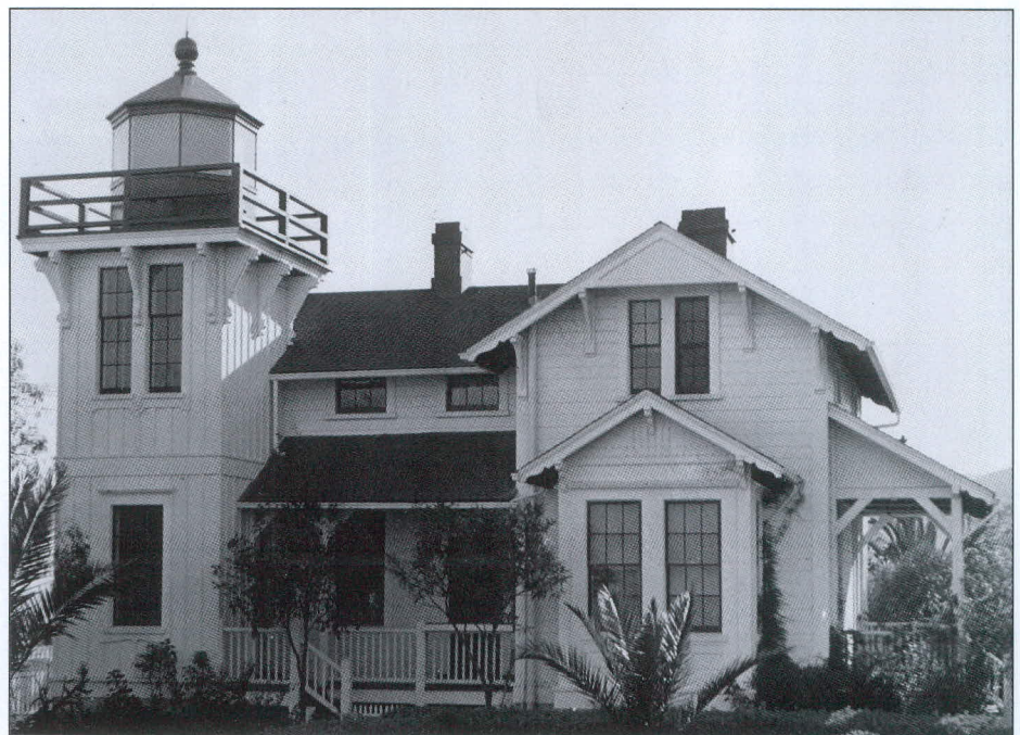
The keeper's house at Ballast Point with tower attached. This building, constructed in 1890, is a duplicate of lighthouses constructed at San Luis Obispo, CA and Table Bluff, CA. The lantern room contained a fixed 5th Order lens. The entire station was razed in 1961. Radford Franke photograph.
